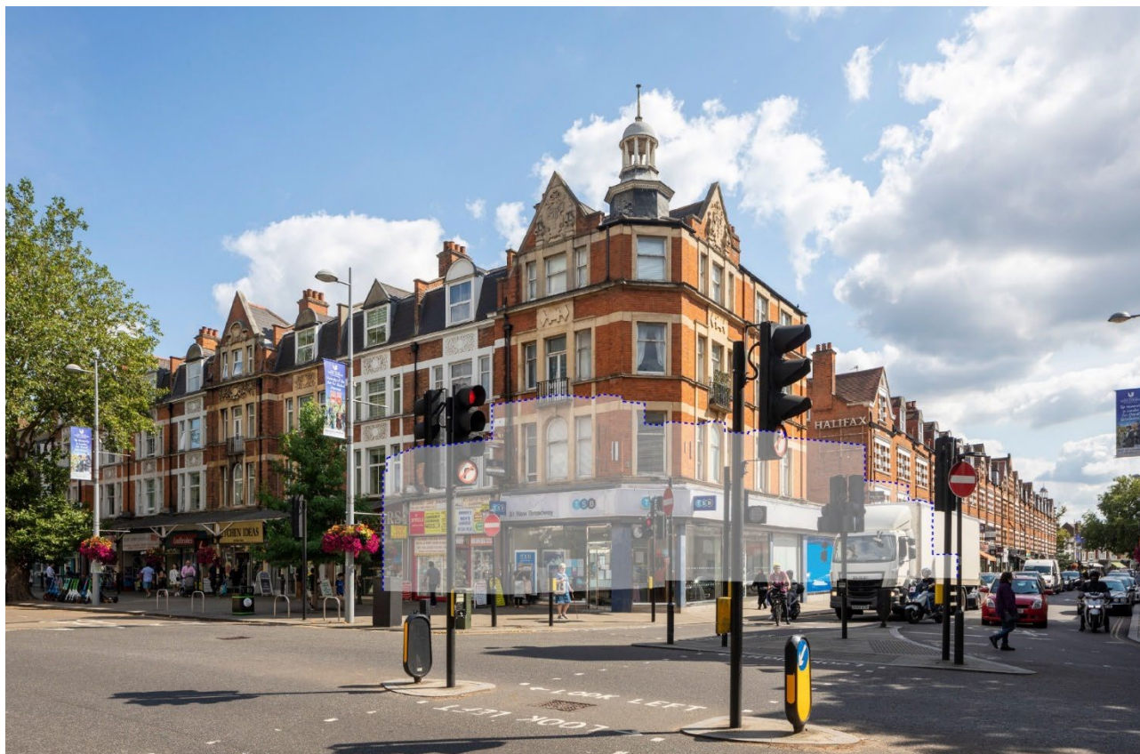
Figure 26: View of proposed development at the New Broadway and Bond Street junction
